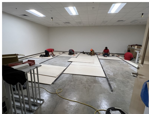
SpaceSaver work crews installing the subfloor.
