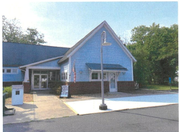
Progress has been made on improving the accessibility into the Northampton Free Library. Pictured here is the new cement pad that makes for a smoother, safer entrance and usable outdoor space.
