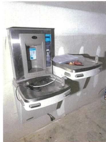
The grant funded water cooler with a bottle filler will be more sanitary and great for tourists and walkers.
