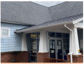
A gutter and flashing was installed to mitigate water damage to the siding.
