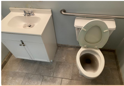
Black silt was in the bathroom water due to lack of use and old pipes.
