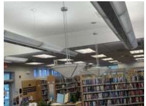
Attractive fixtures can turn out to be expensive to repair and not energy efficient.
