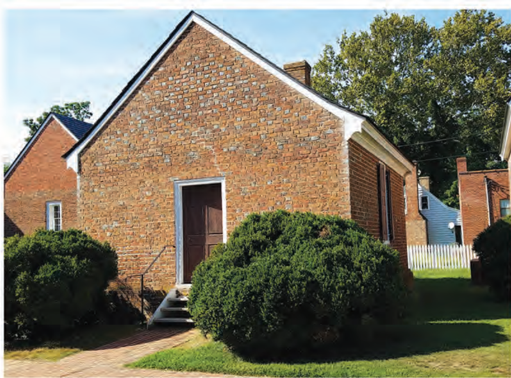
A photograph of the historic Northampton Circuit Clerk's office today. Photo courtesy Jenean Hall.
